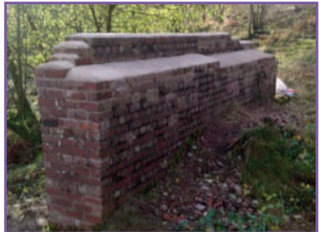
Image: The restored wall Photo credit: Shane Kelleher
