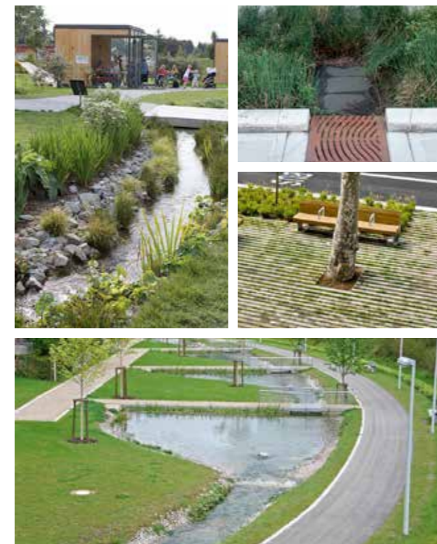
Figure CP.20. Example of surface run-off treatment
