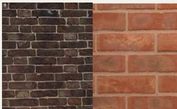
RED BRICK Flemish and stretcher bond
