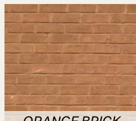
ORANGE BRICK stretcher bond
