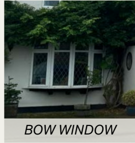
SIDE HUNG with glazing bars
