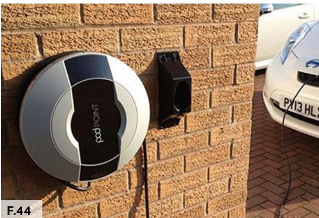
Figure 44: Home electric vehicles charging point
