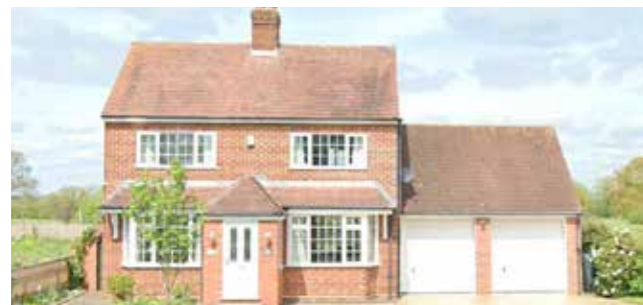
Figure VA.37. Windows arrangement in village area
