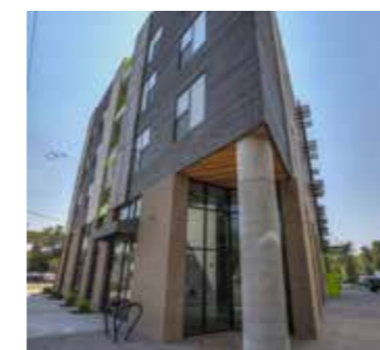
Figure CC.55. Higher ceiling at the ground floor
