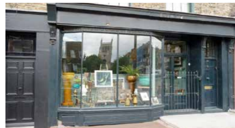
Figure CC.43. Painted timber shop front
