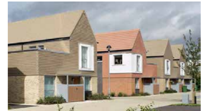
Figure SU.17. Housing cycle storage
