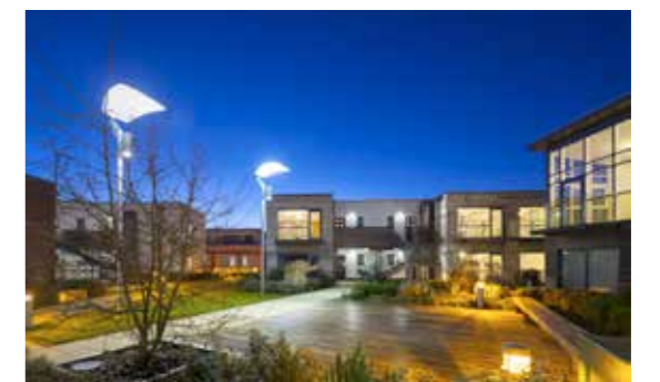
Figure SU.80. Carefully integrated lighting creates safe and usable public spaces.
