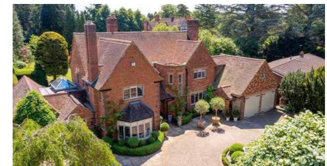
Figure VA.14. Garage in Little Aston
