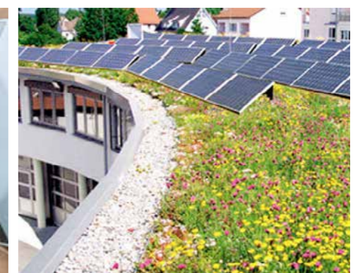
Figure EA.32. Solar Photovoltaic Panels
