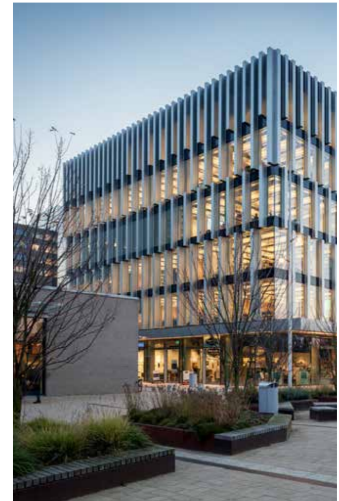
Figure EA.21. Example of offices
