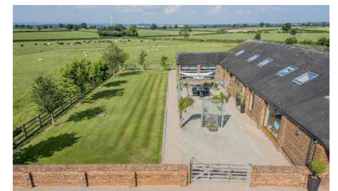
Figure RA.12. An example of agriculture building in rural area
