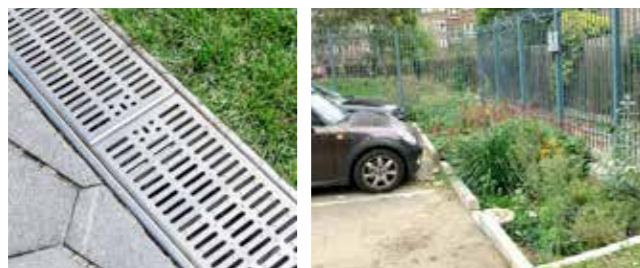
Figure VA.23. Surface Water Drainage
