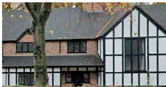
Figure VA.53. Different window types in village areas in Lichfield
