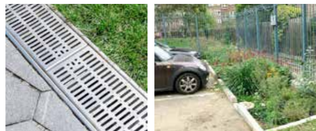
Figure SU.33. Surface Water Drainage Figure SU.34. Intervals to allow water into rain garden
