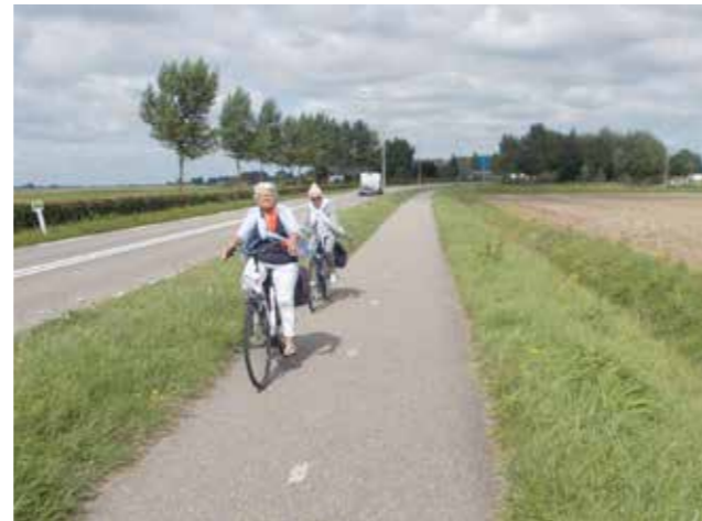
Figure RA.1. Road with cycle lane in rural area
