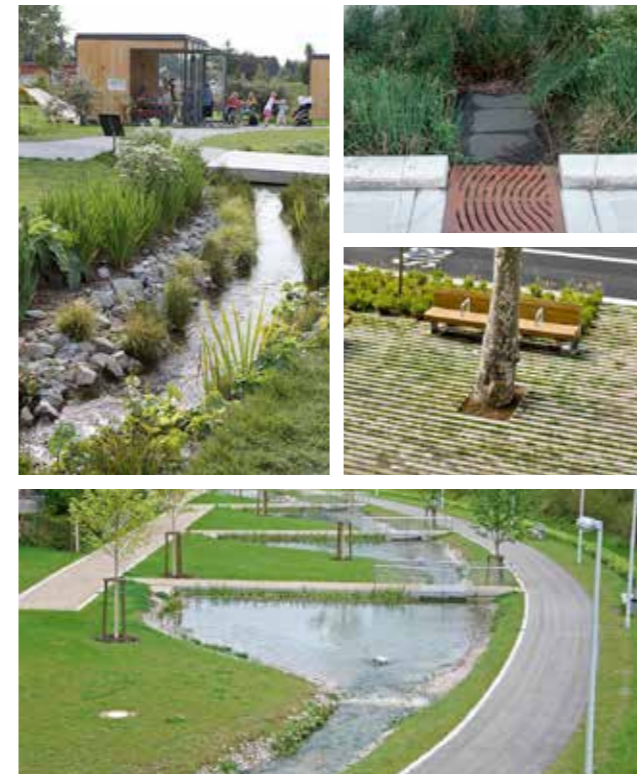
Figure CP.20. Example of surface run-off treatment
