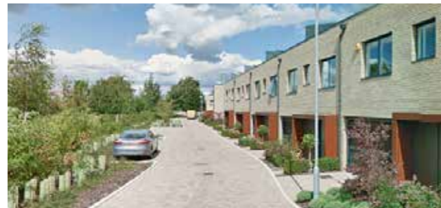
Figure SU.1. Examples of street design providing easy access and movement for all users that encourages walking, cycling, play, and social interaction.
