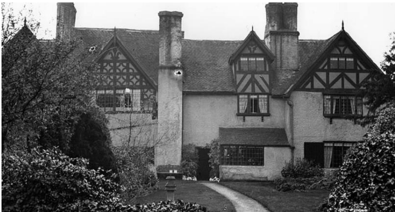
ii Handsacre Hall before demolition
