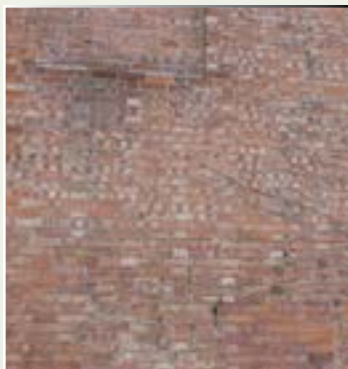
Victorian Brick work
