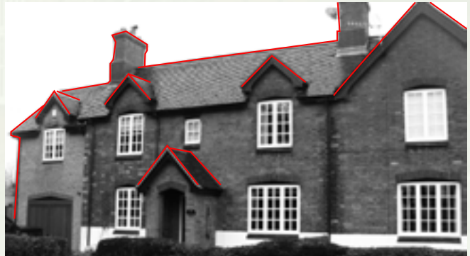
(Figure 31: Victorian Functional Roofscape)
