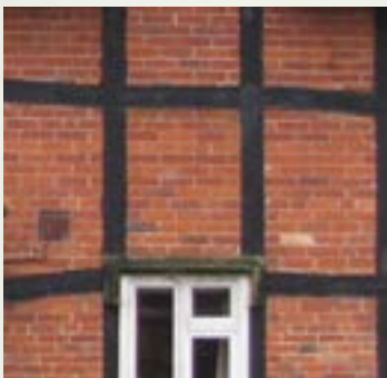
Brick infill with painted timber frame
