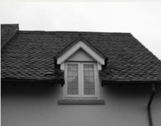
(Figure 16: mixed shingle tiled roof)
