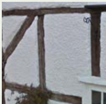
pebble dash infill on timber frame
