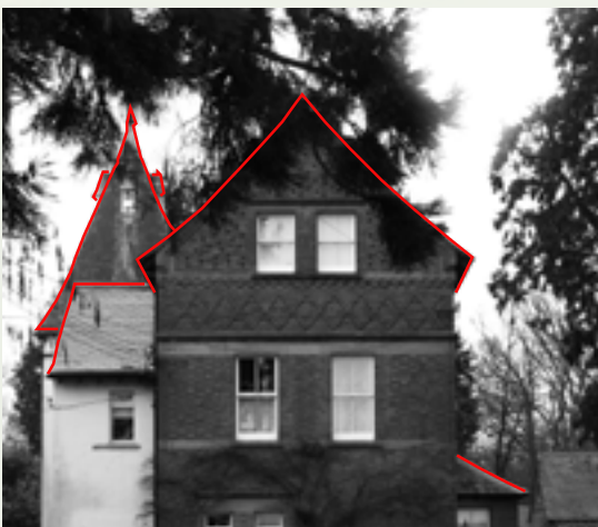
(Figure 32: Gothic Revival Roofscape)
