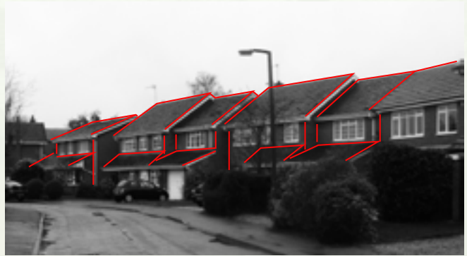
(Figure 29: 1970's residential Roofscape)
