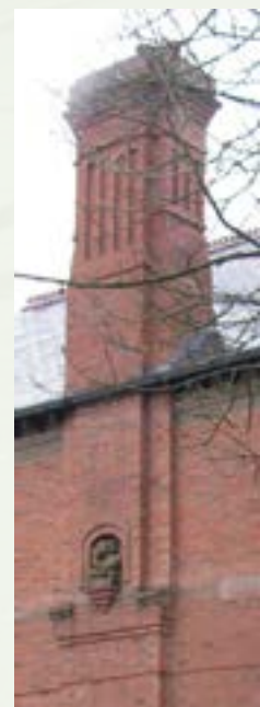
(Figure 13: Gothic Revival Chimney Stack)
