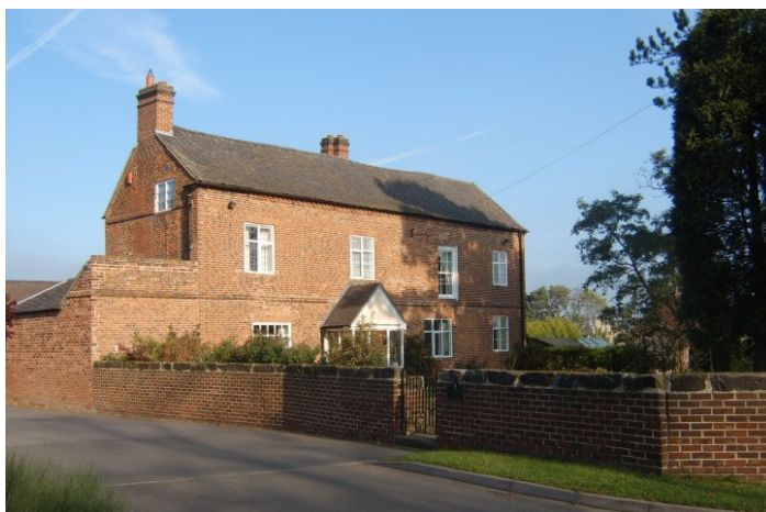
Picture 4.2 Listed Building, Main Street
