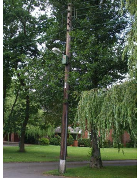
Picture 9.8 A street light on a telegraph pole minimises street clutter
