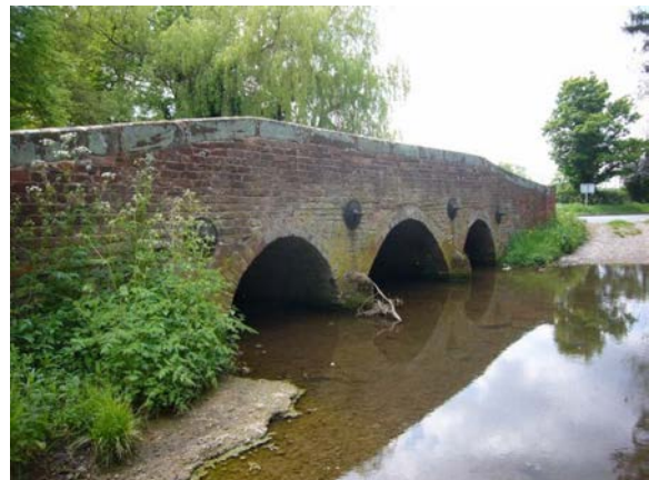
Picture 5.7 Bridge over Moreton Brook
