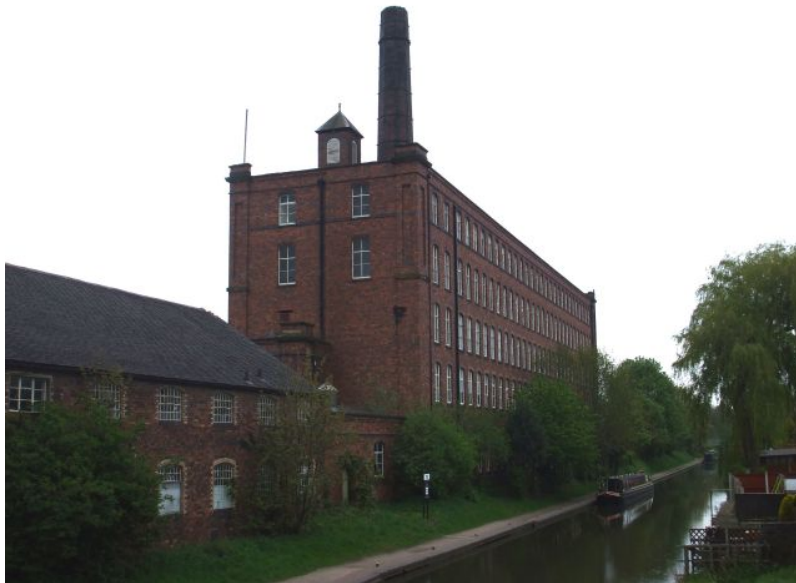
Picture 2.5 Tolsons Mill
