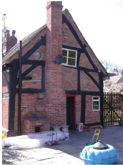
Picture 6.2 17th century timber framing in Park Lane
