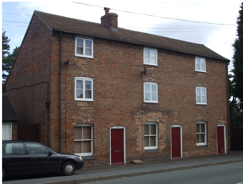
Picture 6.1 110-114 Lichfield Street, traditionally constructed housing c1790
