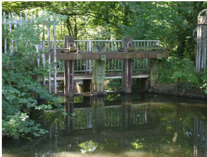
Picture 4.1 Sluice gate at west end of Mill Pool
