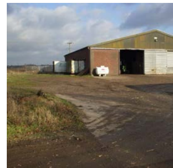
Picture 8.3 Building at Fishpits
