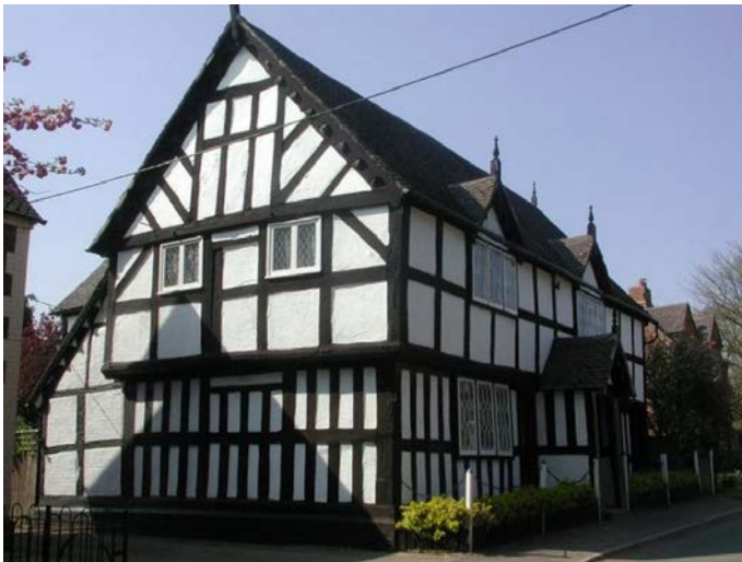
Picture 5.1 The Manor House
