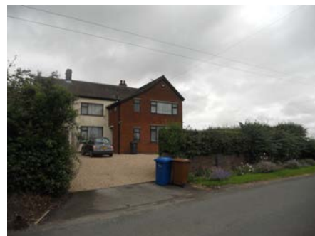
Picture 8.3 Rendered finish and brick exterior on Main Road.
