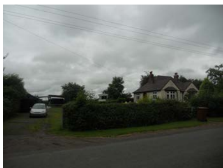
Picture 8.4 Rendered finish exterior on Main Road.
