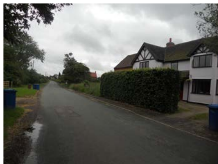
Picture 8.2 Rendered finish exterior on Main Road.
