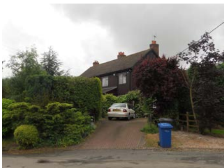
Picture 8.1 wooden panelling exterior on Syerscote Lane.
