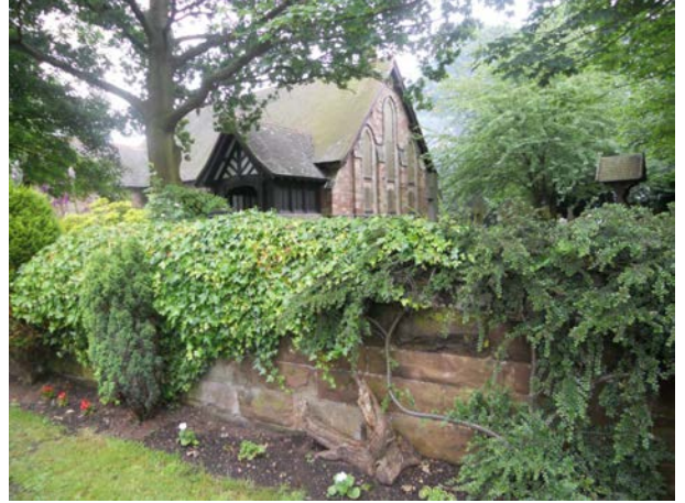
Picture 7.2 Traditional stone wall defining the boundary to the Church.
