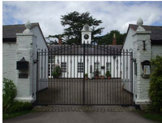
Picture 6.2 Painted brickwork and a slate roof
