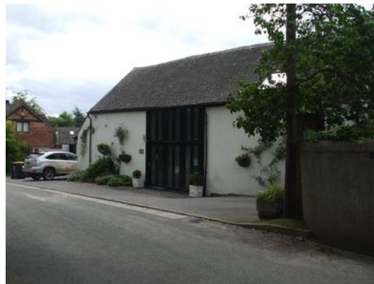
Picture 6.4 Rendered walls and a clay tile roof
