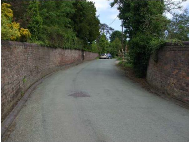
Picture 4.3 General view up School Lane framed on both sides by high brick walls and mature trees
