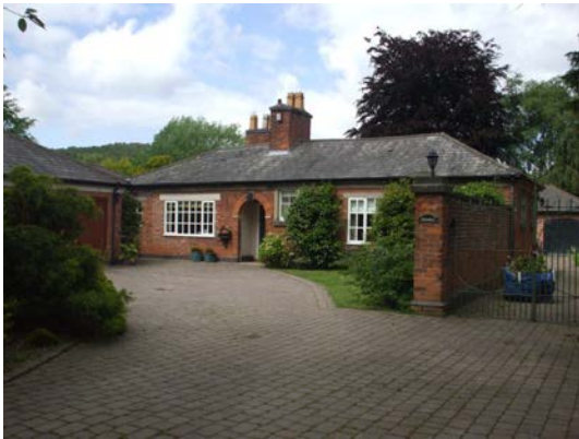
Picture 6.1 Red brick with slate roof - this building was formerly part of Hints Hall
