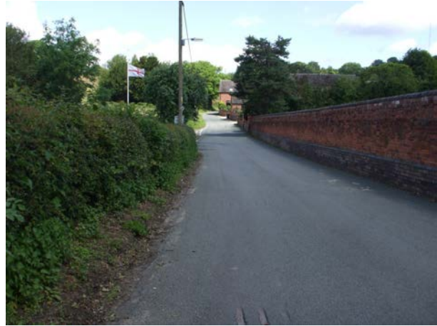
Picture 4.4 General view up School Lane with Manor Farm visible in the distance
