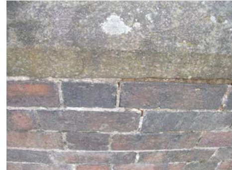
Picture 6.7 Accommodation bridges are of brick, with a stone finish.
