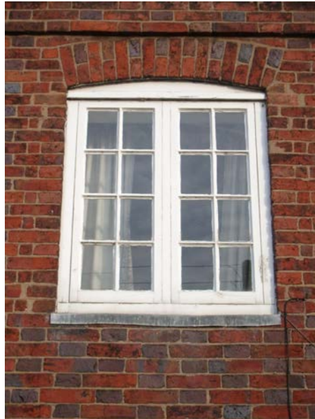
Picture 6.9 Traditional timber frame windows remain on the majority of the historic buildings
