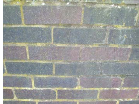
Picture 6.6 Boundary walls may be made of blue brick
