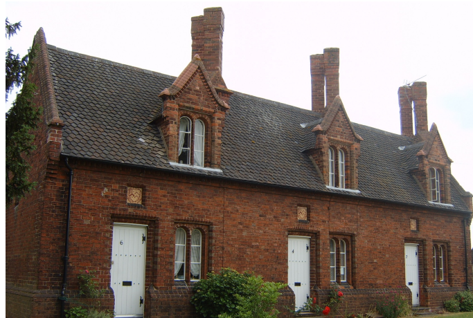
Picture 4.5 Almshouses, corner of Manor Rd and Yoxall Rd
