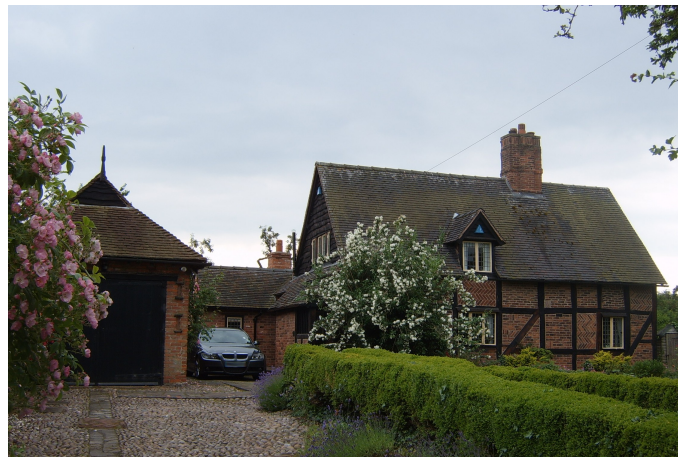
Picture 4.6 Listed building, Manor Road
