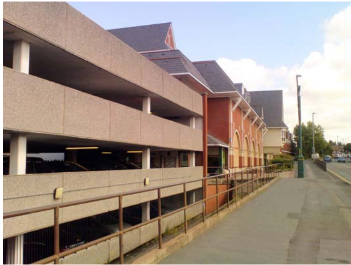
Picture 16.37 Birmingham Road showing lack of active frontages
