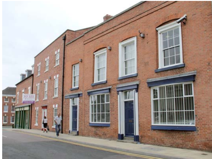
Picture 16.8 Office buildings along Sandford Street
