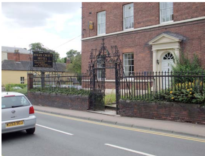
Picture 16.43 Front boundary wall and ornate wrought iron railings to the Angel Croft Hotel
