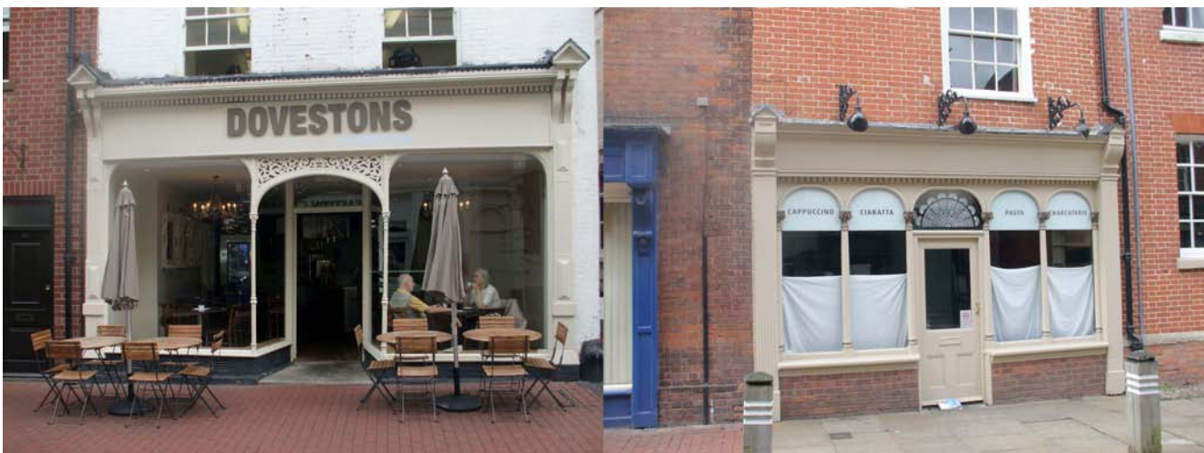
Picture 16.7 Historic shopfronts at numbers 16 and 27 Bird Street
