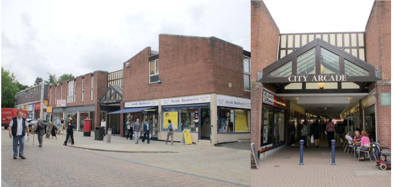
Picture 16.20 1960's development on the corner of Bird Street and Bore Street
