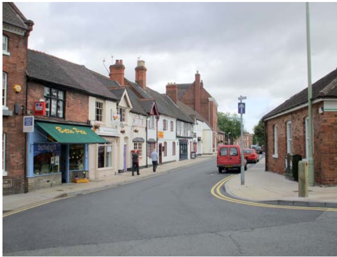
Picture 16.25 Timber framed buildings along Lombard Street with later brick and render facades
