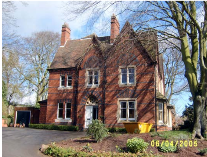
Picture 8.4 Mid-Victorian house
