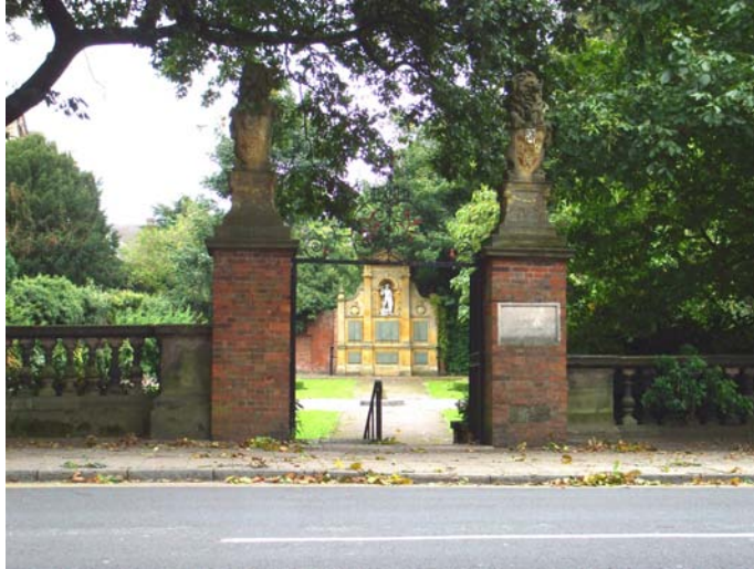
Picture 14.11 The gatepiers and gates to the Memorial Gardens that would be restored as part of the Lottery bid.
