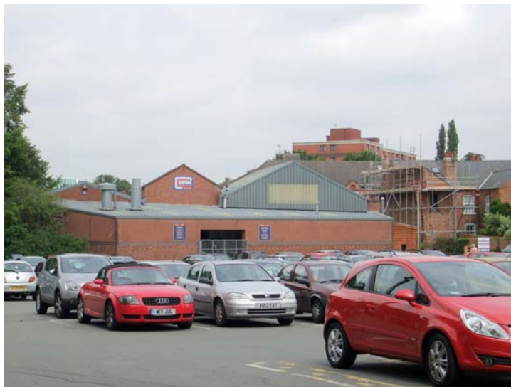
Picture 14.26 Poor view across Friary Car Park
