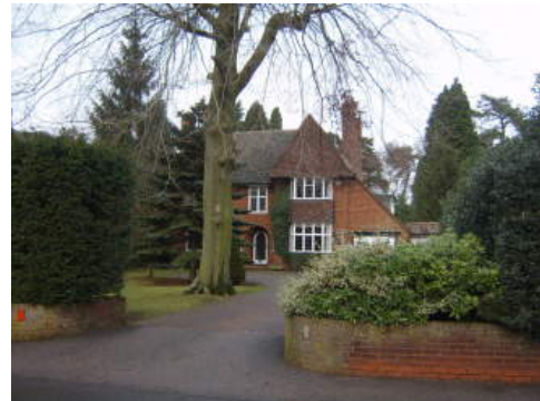
Picture 4.6 Hardwick Road. An example of some typical boundary treatments
