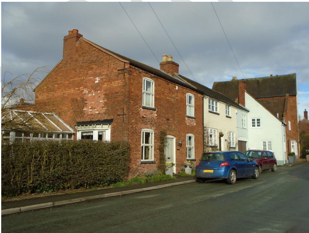
View of properties on Watling Street
