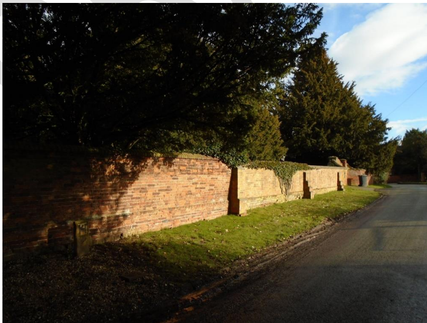
Boundary wall of Wall House, Green Lane
