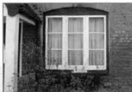
Detail of window at 1 Main Street
