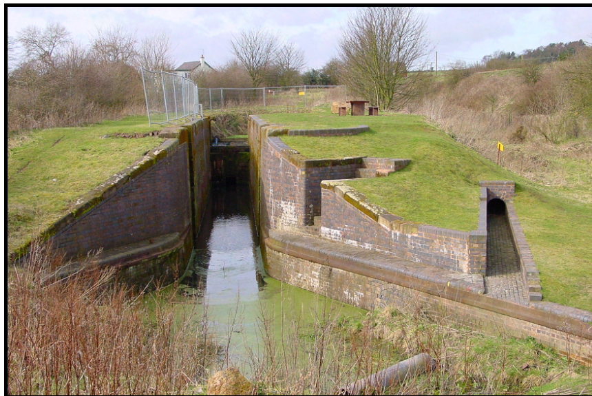
Lock 18, restored by the Trust, awaiting gates, paddle gear and boats.
