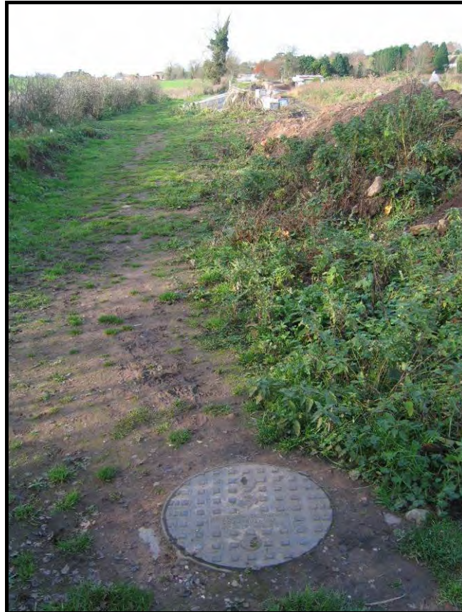
Manhole on culverted land drain, looking towards Lock 26
