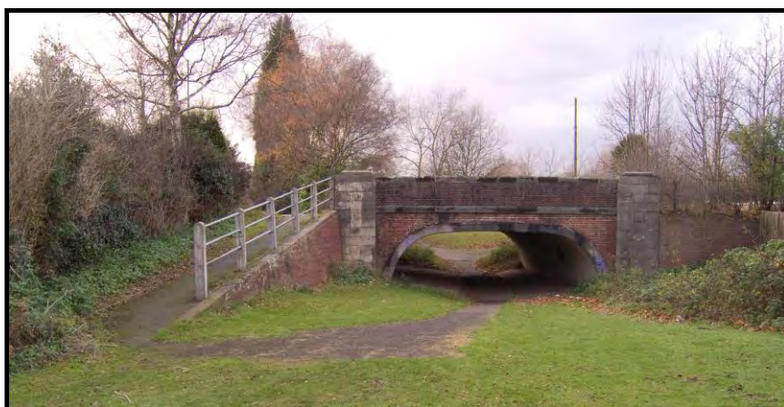
London Road Bridge from the east.
