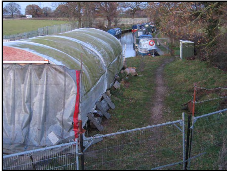
LCC moorings from Cappers Bridge, showing the covered slipway
