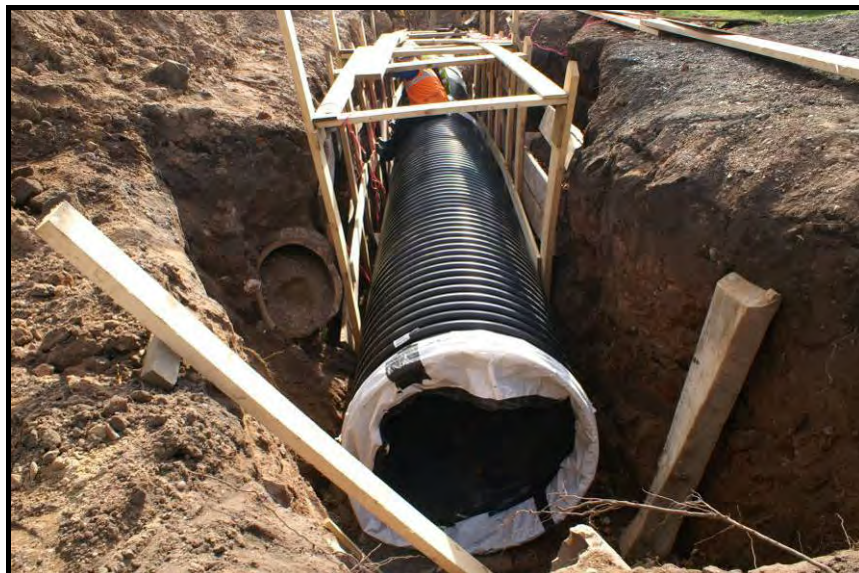
Trust members installing new bywash culvert to Lock 25, early 2009
