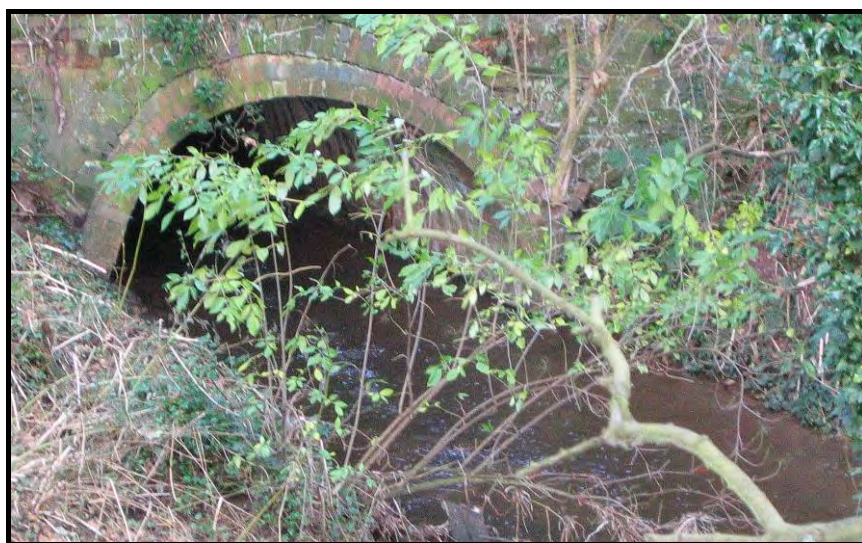
Culvert carrying Pipehill Brook under the canal embankment.
