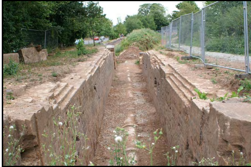
Lock 24, whilst uncovered for investigation, looking downstream.
