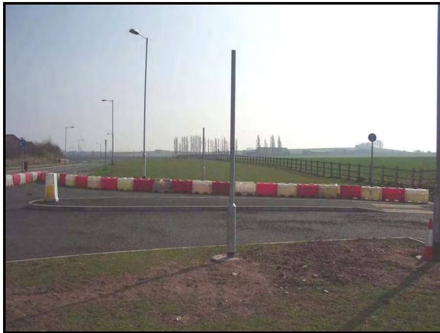
The site for Claypit Lane Bridge, looking east (downhill) towards the proposed Lock 19 to Lock 21 flight.
