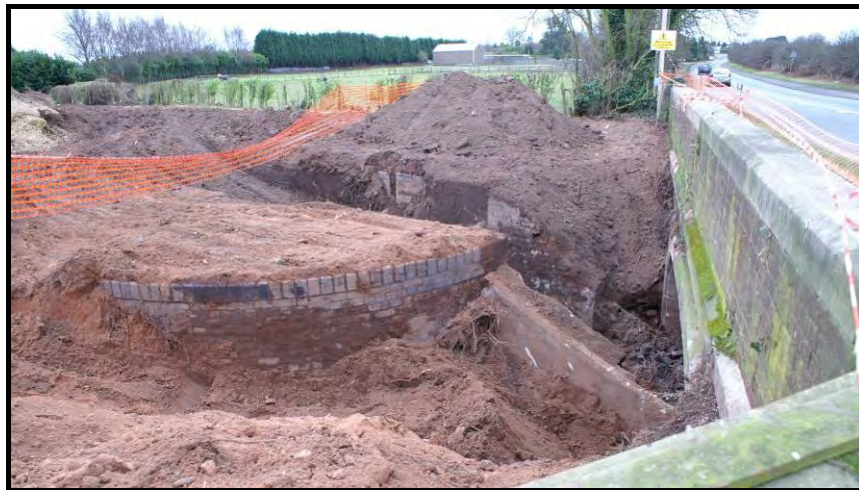
Lock 11 exposed recently during works undertaken by Staffordshire Highways 39
