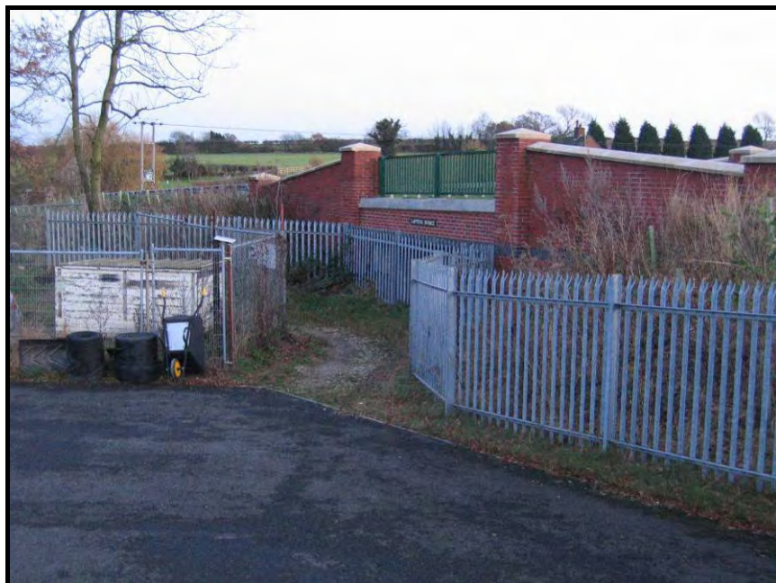
Cappers Bridge from Cruising Club car park / service yard
