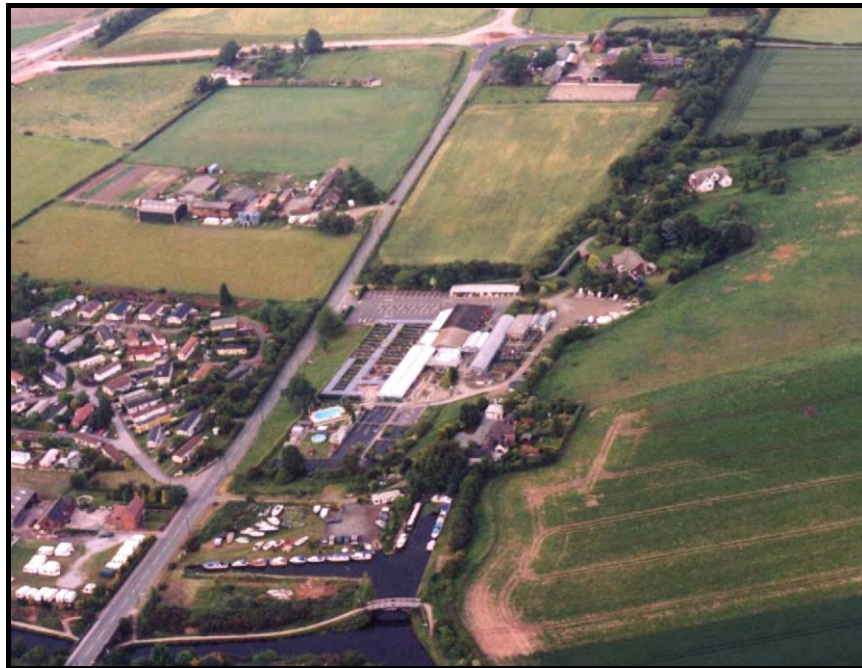
Aerial photo of the Ogleby Locks Flight, running centre bottom to top right on the picture. Ogleby Junction is at the bottom, Barracks Lane and Lock 6 right at the top. 45
