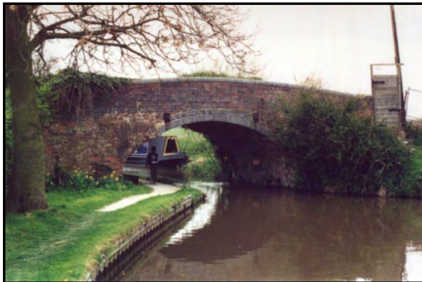
Watery Lane Bridge 18
