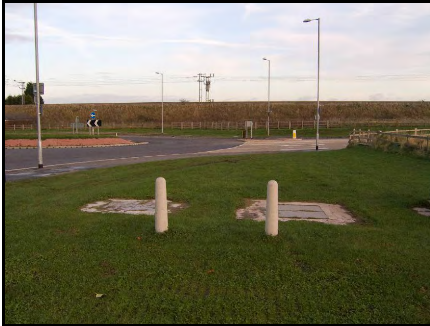
Looking east across the new Birmingham Road – Southern Bypass roundabout, along the line of the Birmingham Road Culvert, to the approximate location for the railway crossing (under the catenary posts)
