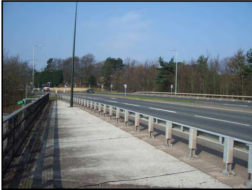
Looking west along the A51 Tamworth Road. The proposed canal culvert will cross roughly between the two galvanised street lights in the middle distance.
