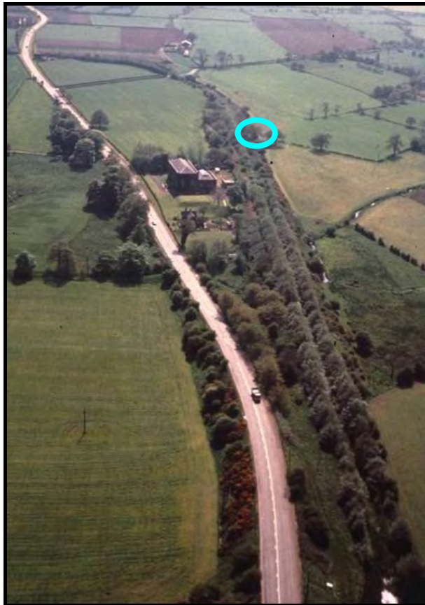
Aerial view of Pipehill Embankment and Pumping Station from above Pipehill Bridge – winding hole location circled.
