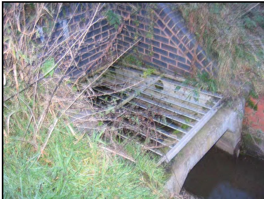
Darnford Brook Culvert – Downstream Headwall
