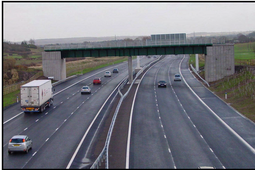
The M6 (Toll) Aqueduct, seen from the A5, looking south east. The approach embankment on the left gives an idea of the original canal level below Lock 8.
