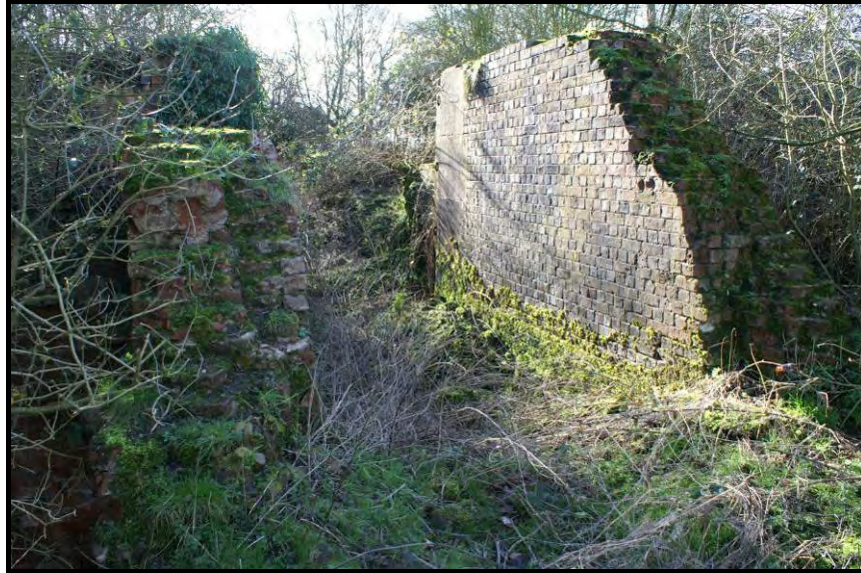
Remains of Lock 29, to be left in current state in offside woodland 22
