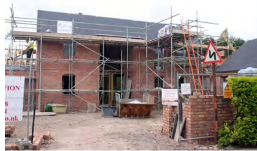
Dwelling under construction, Mill End Lane
