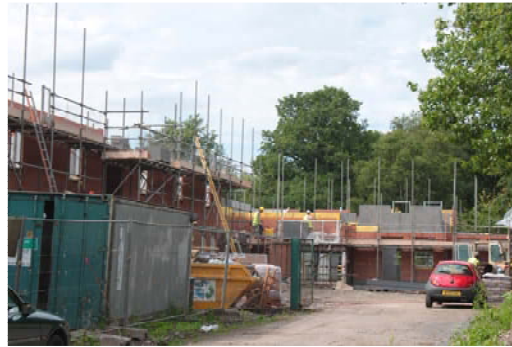
Housing under construction at Lynn Lane Shenstone
