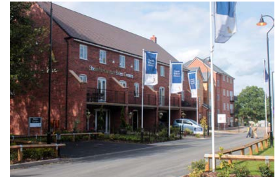
New housing at Fazeley
