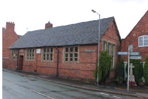
Old school building on Church Street
