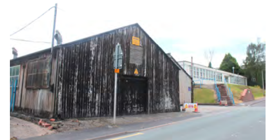
Part of Ideal Standard works, Old Rd.
