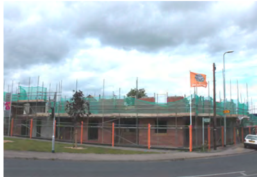
Housing under construction at Handsacre
