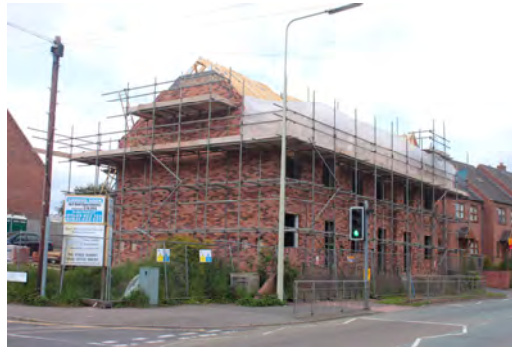
Housing under construction, Handsacre
