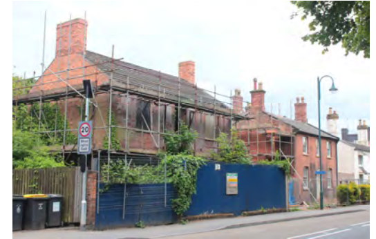
Houses on Coleshill Street: scaffolding
