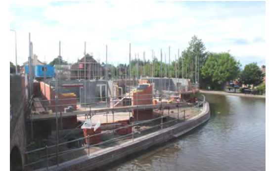
Development under construction, the Boathouse, Fazeley
