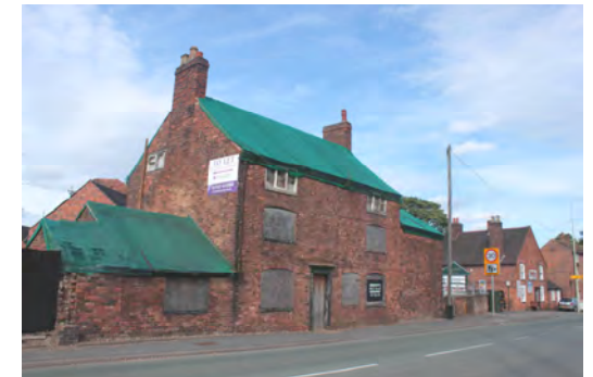
Empty building Lichfield Street
