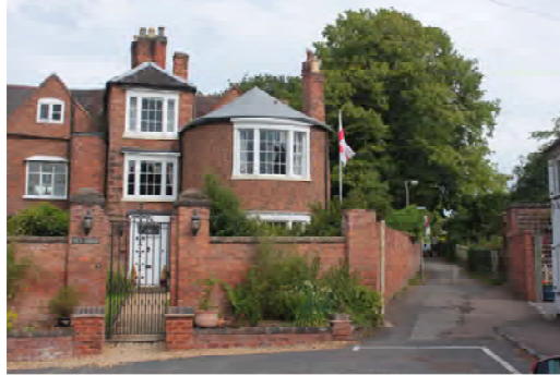
Part of the Conservation Area, Main St.
