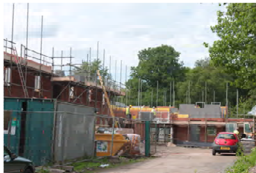
Housing under construction, Lynn Lane
