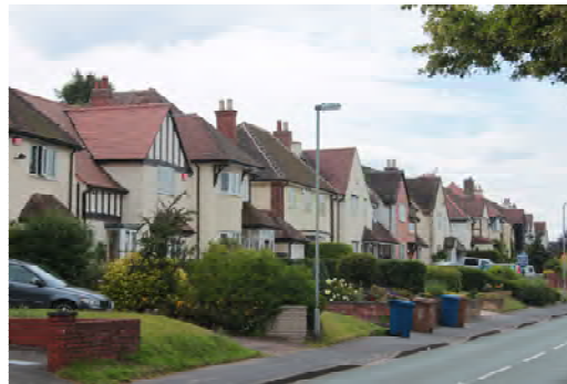
Housing on Little Aston Lane
